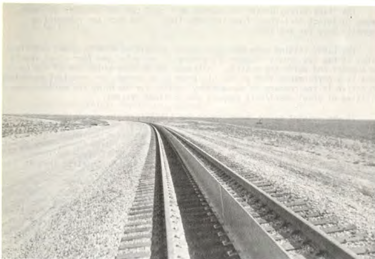
View of LIMRV Test Track Showing Aluminum Reaction Rail Installed Mid-Way Between the 119 lb. Conventional Running Rails. Location is on 0°-26' Curve Having 8° of Superelevation.
