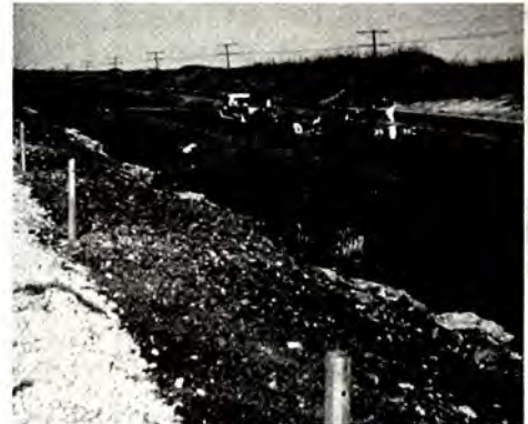
INSTALLATION OF VERTICAL DISPLACEMENT TRANSDUCERS AT ONE OF NINE MAIN ARRAY INSTRUMENTATION LOCATIONS.
