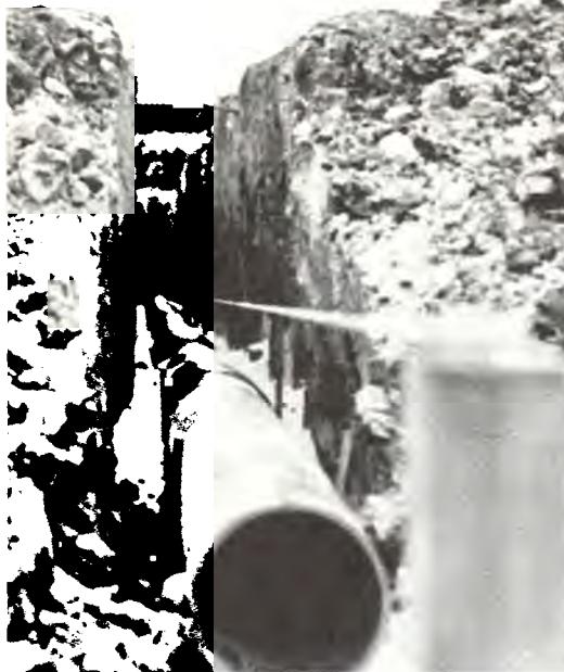
ENBANKMENT HORIZONTAL DISPLACEMENT TRANSDUCER REFERENCE TUBE INSTALLED PRIOR TO BACKFILLING.
