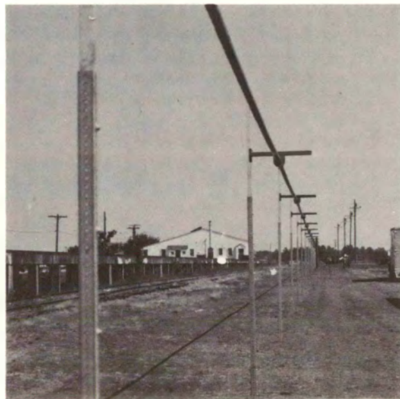
Figure 40. Communication Cable Mounted on Metal Poles and Supported with Wooden Clamps at Ft. Devens, Mass.
