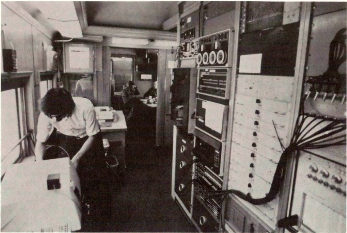
Figure 31. Data Recording System on an Operating Train.
