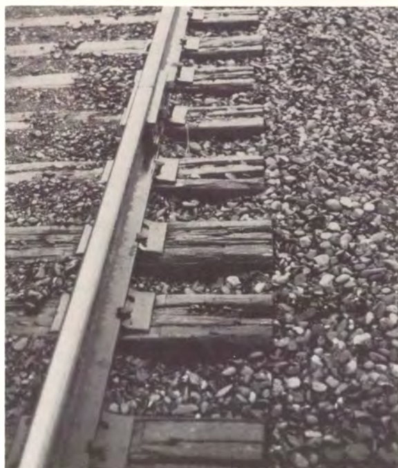
Figure 10. Alaska Railroad Ties "Spike-killed" by Frequent Realignment.
