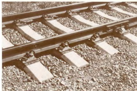
Figure 30. Pandrol Fasteners attached to Adjustable Base Plates in the Montana Test of the Alaska Railroad. (railends have now been welded).
