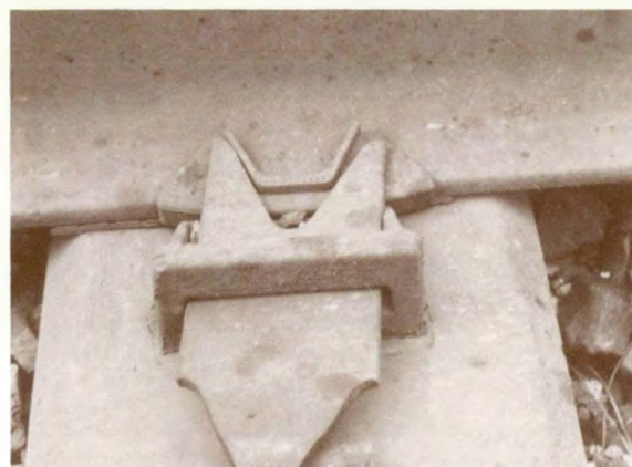
Figure 33. Pad Displacement and Skewed Rail Fastener, Chessie Test at Lorraine.
