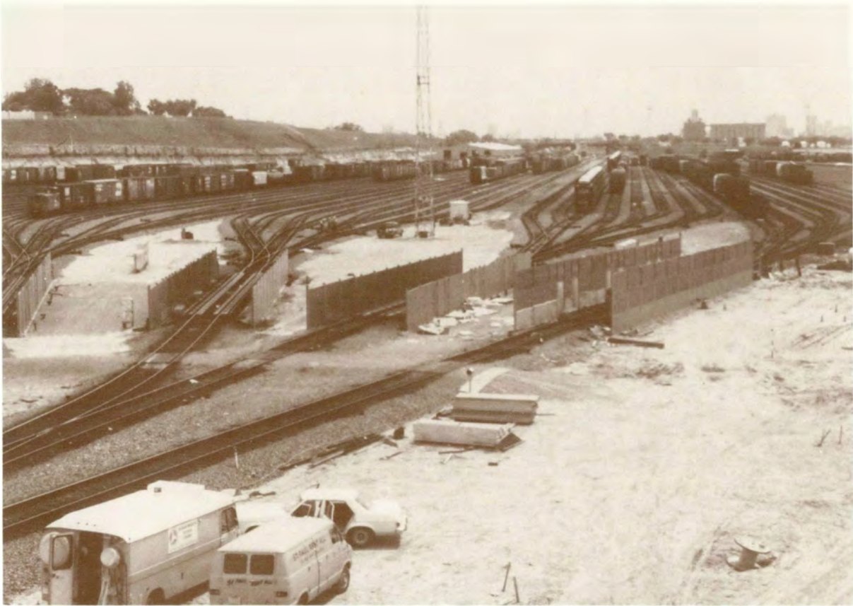
Figure 3. View of Burlington Northern's Northtown Yard at Fridley, Minn. In the foreground can be seen acoustic barriers used to attenuate the noise generated by the master retarders when controlling railcar rolling speed. Project is to evaluate the effectiveness of different acoustic barriers.
